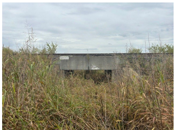
Box culvert under railway
