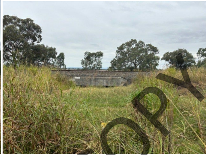
Box culvert under railway
